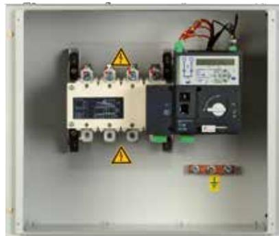
**Standard offer includes Bottom cable entry. Top cable entry is offered as an option.**
